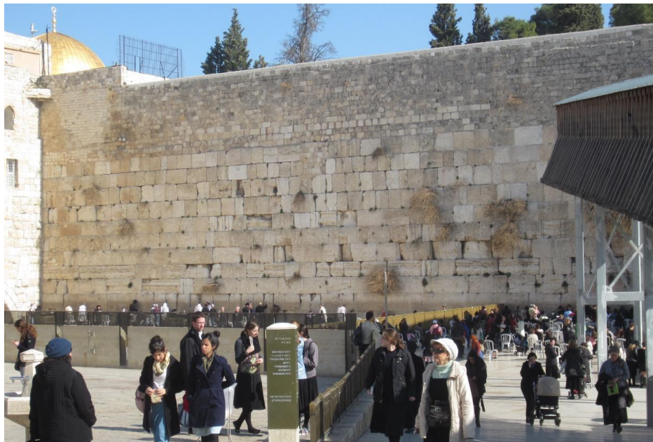
The Western Wall of the Temple Mount: the only remains of the original retaining wall. Photo by Victoria Larson.
